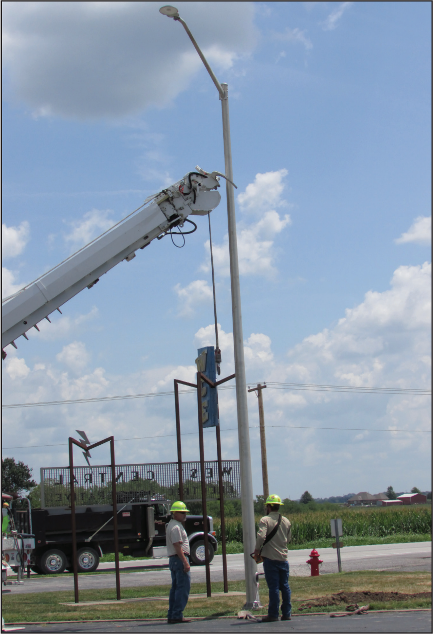
CONTINUED IMPROVEMENTS...Work continues on updates at the WCE headquarters building in Higginsville. (Top photo) WCE lineman Derek Cole works on getting a new parking lot light connected. (Bottom photo) Eric Wegener and Cole get the new light pole set.
