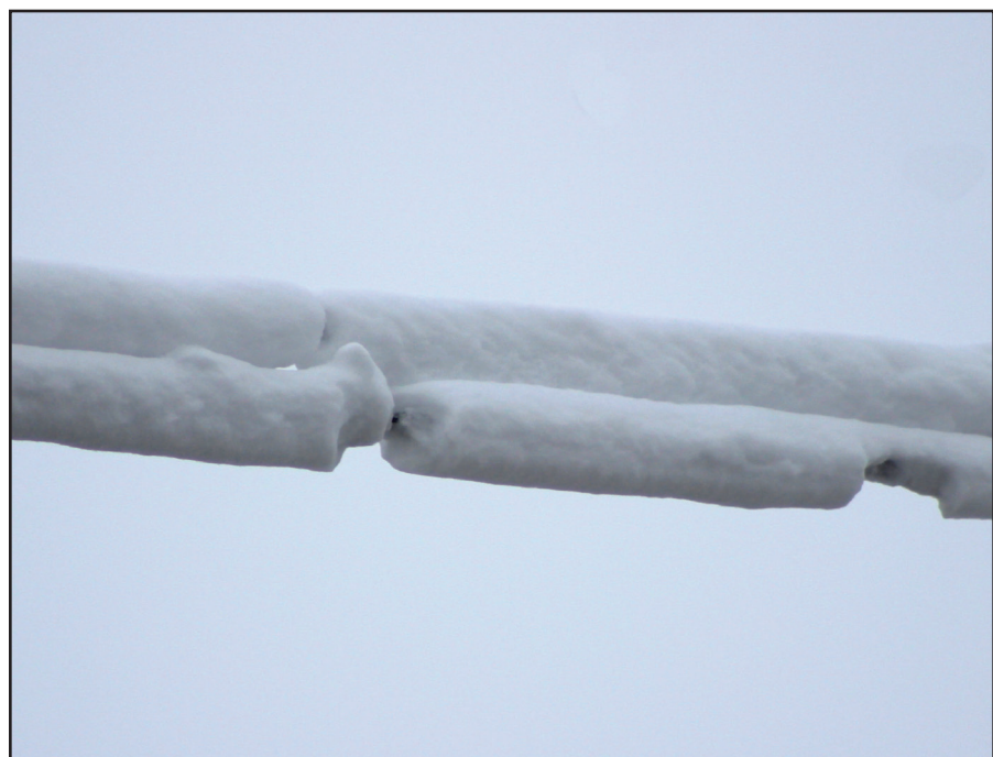
SURROUNDED... Lines were surrounded by snow causing them to sag. Several outages occurred as snow began to fall off lines causing them to "gallop" and slap together.
