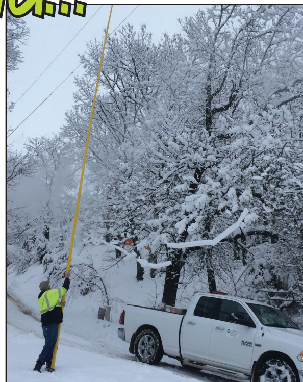
DOWN IT COMES... Linemen spent a lot of time knocking off snow that had accumulated on lines, causing them to sag. Above, serviceman Robert Mlnnis clears a line of snow.
