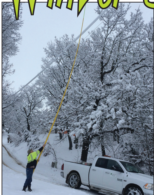
DOWN IT COMES... Linemen spent a lot of time knocking off snow that had accumulated on lines, causing them to sag. Above, serviceman Robert Mlnnis clears a line of snow.
