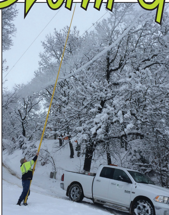
DOWN IT COMES... Linemen spent a lot of time knocking off snow that had accumulated on lines, causing them to sag. Above, serviceman Robert Mlnnis clears a line of snow.
